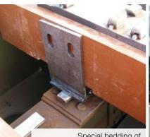
Special bedding of FFU synthetic sleeper on open steel support structure
