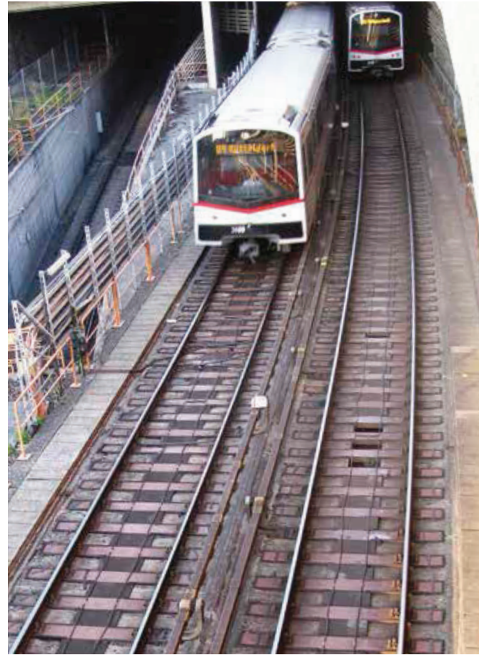
100 mm deep FFU sleepers have been used on several sections of Wien U-Bahn lines U1 and U4.
