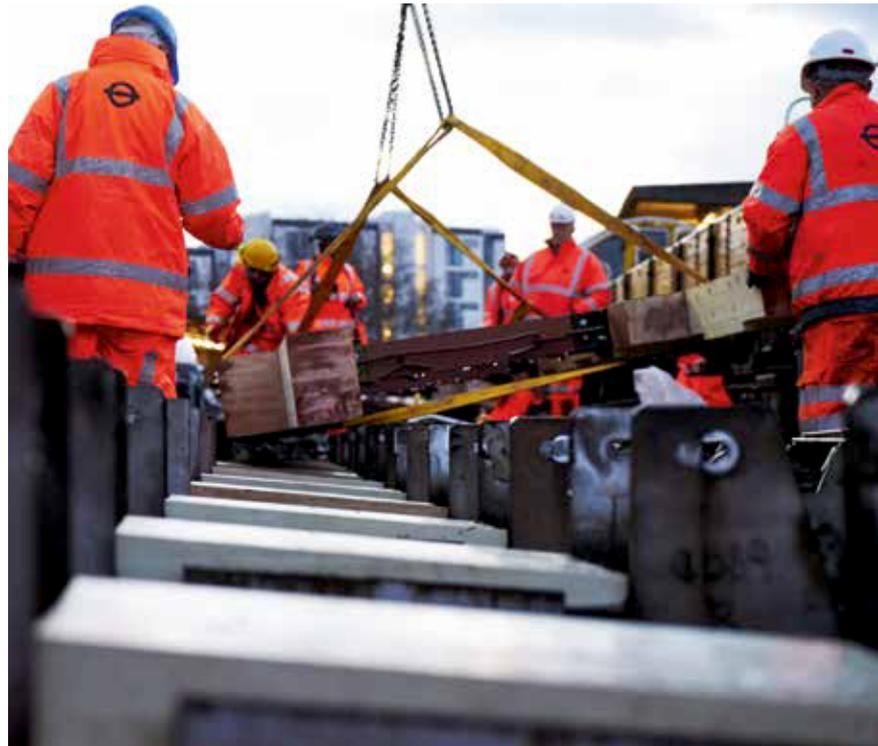
The prefabricated FFU frame is brought in to rest on FFU wedges (above). Work was finished on March 6 (left).
