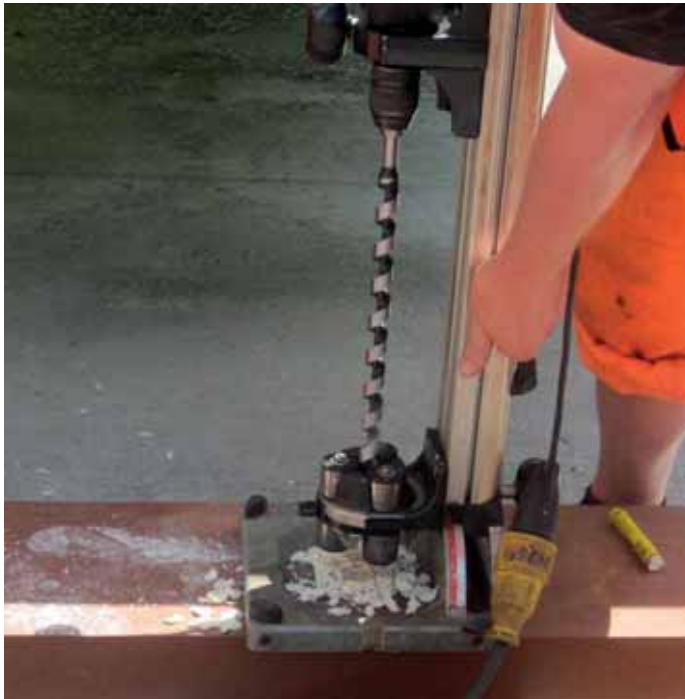
Making bore holes in the synthetic wood sleeper
