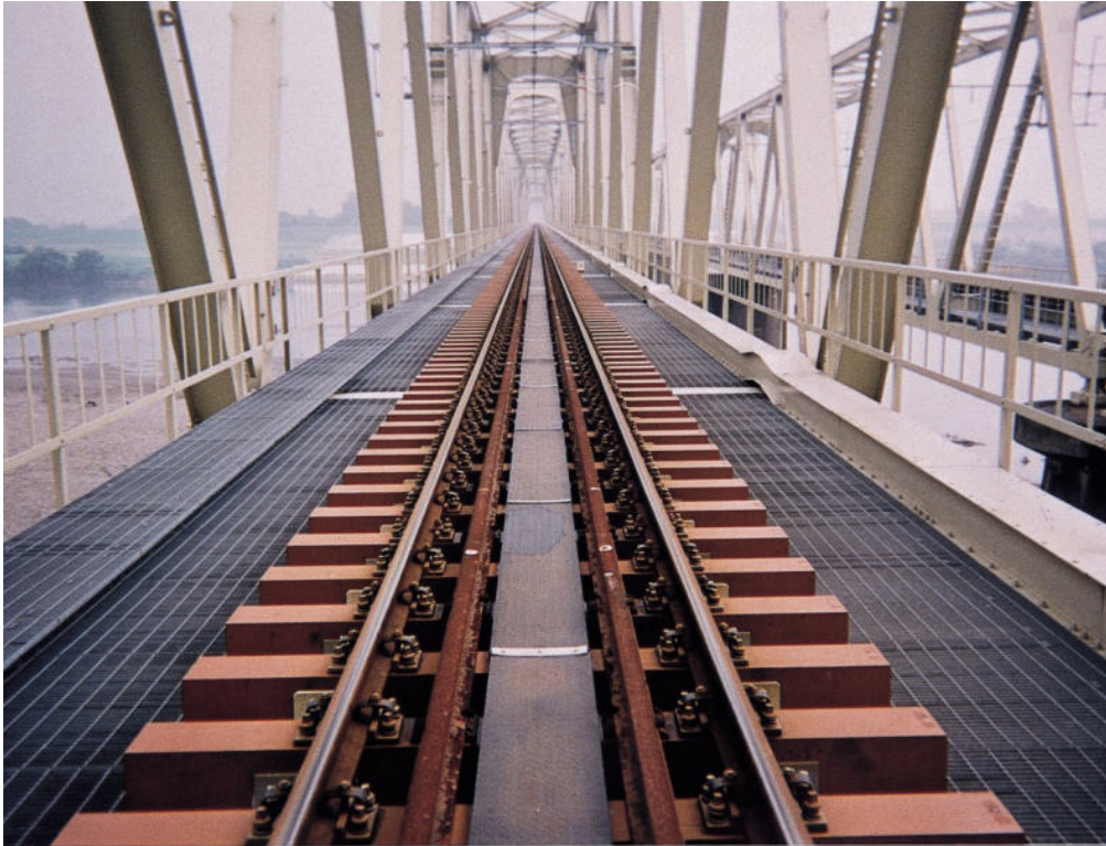
Picture 4: FFU bridge sleepers on Shinkansen track - Japan
