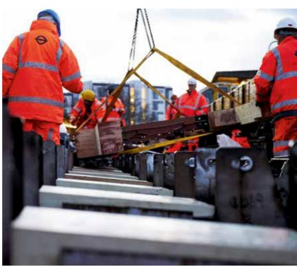
The prefabricated FFU frame is brought in to rest on FFU wedges (above). Work was finished on March 6 (left).
